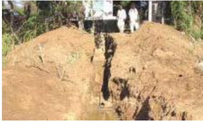
Construction of a subsurface dam
