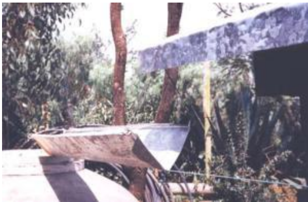
The first gutter laid along a drawn string
