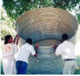
A leaking water tank made of galvanized iron sheets
