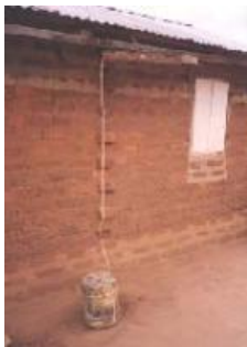
Simple roof catchment
