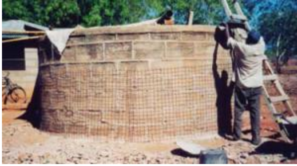
Weld mesh wrapped around a tank.
