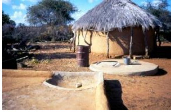
Traditional underground cylindrical water tank in Botswana
