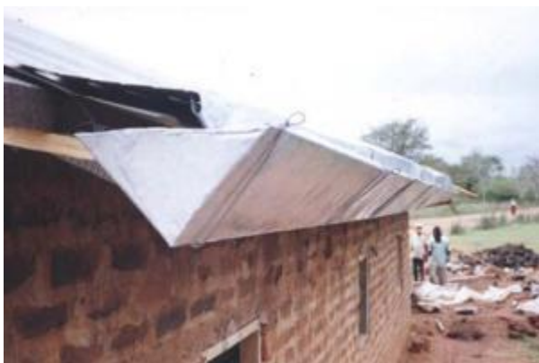
Gutter laid in hangers
