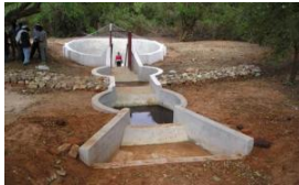
Berkad ground tank in Kenya
