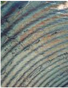
Chicken mesh tied to the interior of a tank
