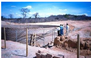
Building a cylindrical water tank in Tanzania
