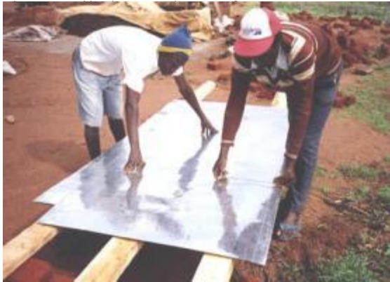
Marking an iron sheet into three stripes with a wire
