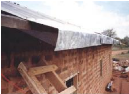
Splash-guard being nailed into a roof
