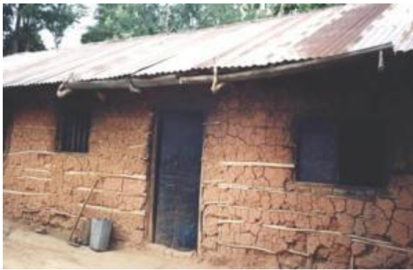
Simple and cheap gutter laid in tree branches
