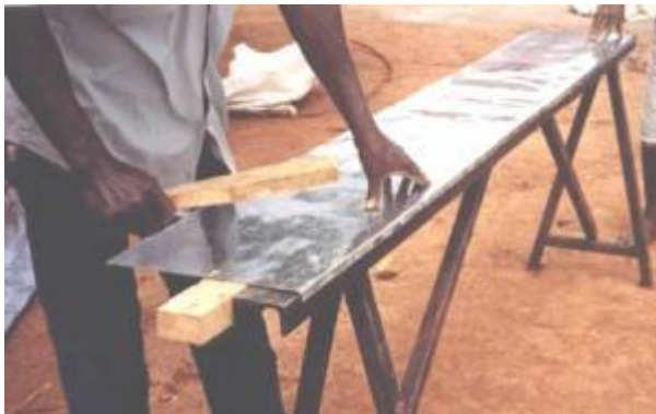
Bending the edge of an iron sheet
