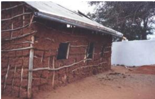
Gutter suspended with a straight slope from a splash-guard nailed onto an uneven roof
