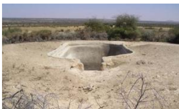
Berkad ground tanks in Somaliland
