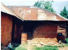
An oil drum used for roof catchment at a rural home
